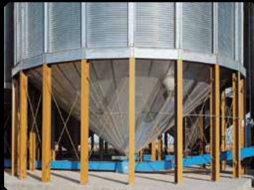
40 DEGREE HOPPER SLOPE
