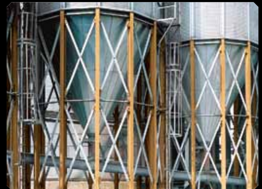
60 DEGREE HOPPER SLOPE
